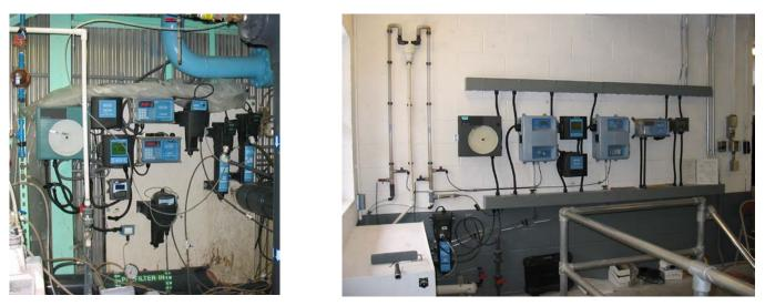
Chaos or control? If you analytical gear installation is a bit of a hodge-podge like the picture on the left, check out what our Timber Line staff helped create for Castle Pines! Wireway is mounted at the top to receive control and power wiring, non-metallic flexduit keeps wires dry, and the lower wireway is off-set from the wall with unistrut to allow the conduit, cables, and drain tubes to exit in an orderly fashion. The operators really like the displays being at eye level!
